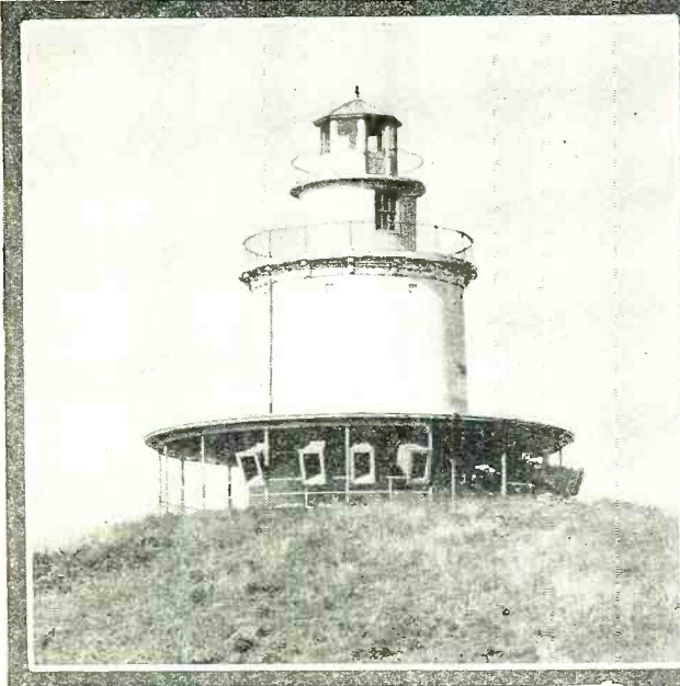
The odd structure above serves, not only as a lighthouse, but also as a community radio loud speaker. It is located at Dartmouth, Mass., where the Round Hills Radio Corporation maintains station WM&F. Around this battery of huge speakers the whole population of the town may gather on pleasant evenings to hear programs reproduced with a volume that fills all outdoors.
