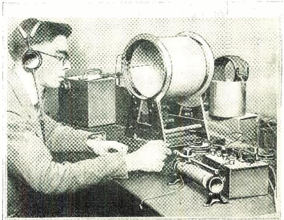
Morris S. Strock making measurements of frequency of the wave of a broadcast station. A large number of wavemeter coils are kept by the Bureau for this special work of checking standard-frequency signals.
